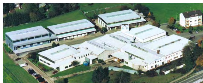
BOSCHERT'S modern plant in Germany's Black Forest region.
